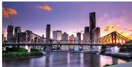
Brisbane City River Story Bridge
